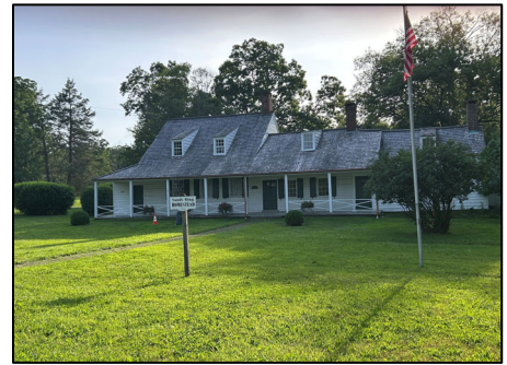
The Sands-Ring Homestead, or Old Homestead, dates back to the 1700’s. This Dutch-colonial style building is one of the oldest in Cornwall and one of the most historic. It was inhabited by the Nathaniel Sands family and their descendants from the early 1750’s until 1907.
